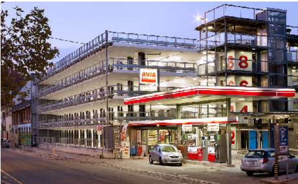
Parkhaus, Sihlquai 41, 8001 Zürich
